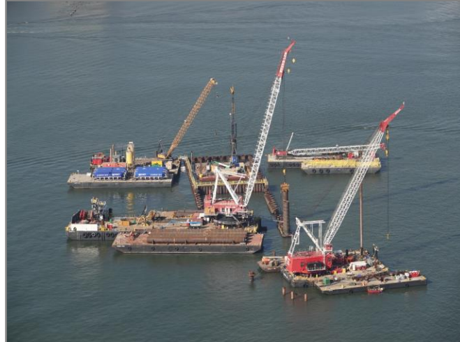
Aerial view of work area location Oct 22 nd , 2024 (looking West)
