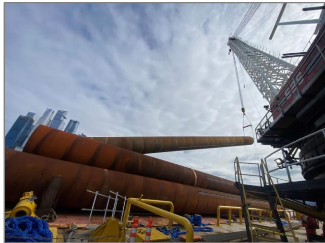
King (Production) Piles being lifted into place Sep 30 th , 2024 (looking East)
