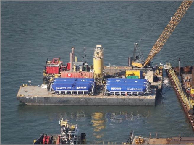
Batching and Dry Binder Storage (Pig) Barges Oct 22 nd , 2024 (looking West)
